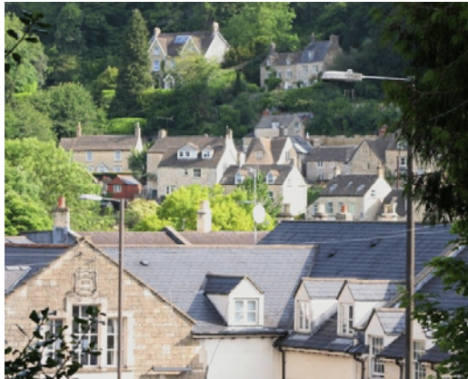
Weavers cottages in Watledge overlooking Nailsworth
